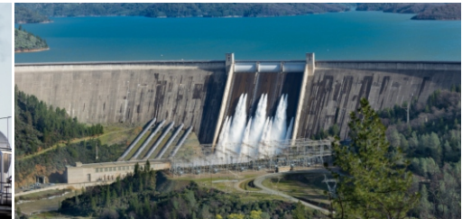
Dam & Hydroelectric Power Plants
